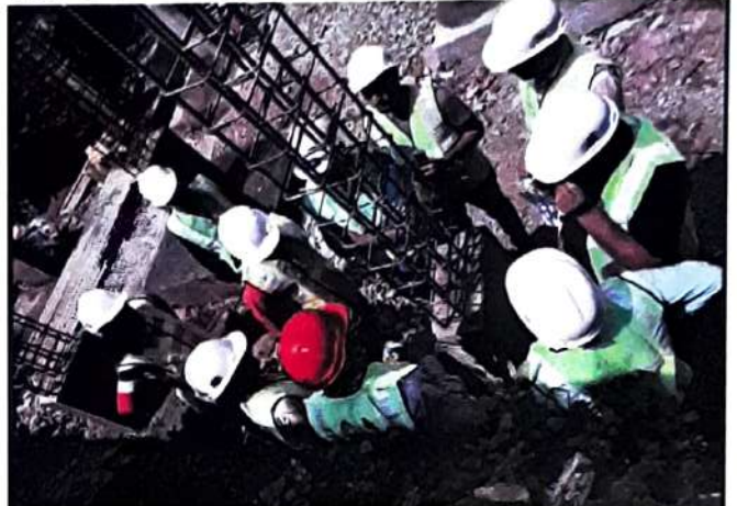
Fig. No. 6 Instructor giving instruction about four major hazards during concreting
