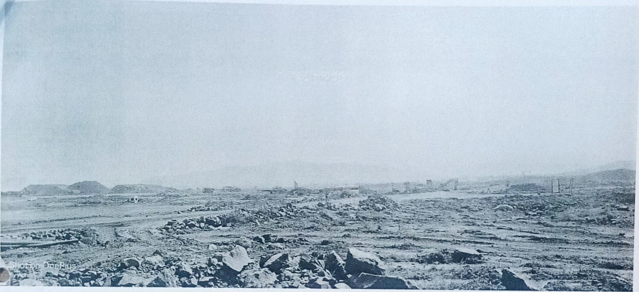
Figure 9: Runway Site before clearing the ground
