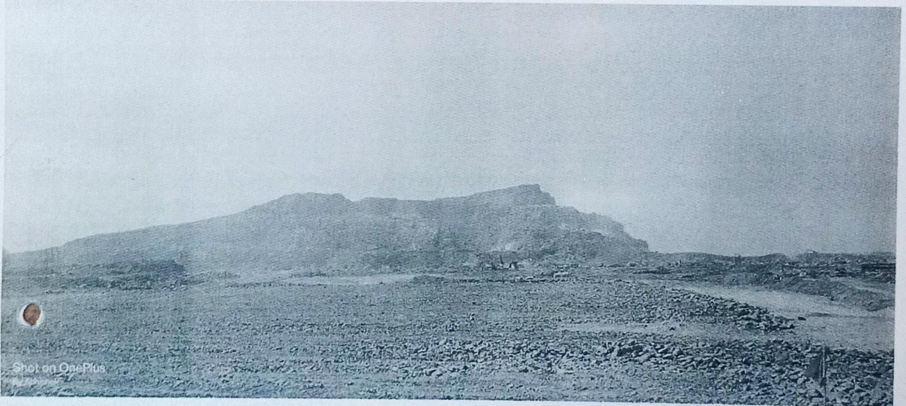
Figure 10: Runway site after clearing the ground
