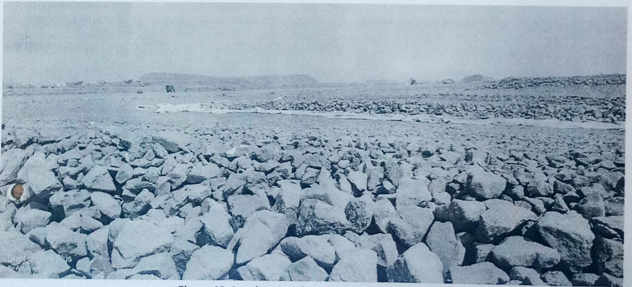
Figure 12: Local material used in construction of runway
